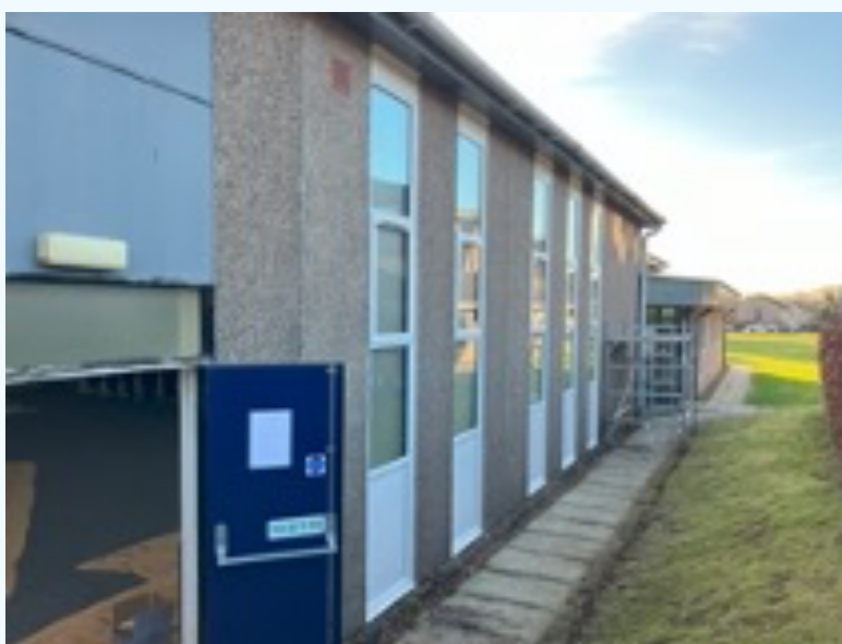
The north wall with new windows in place
